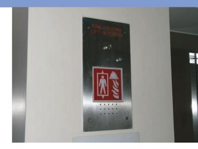
by running two independent, fireresisting circuits via diverse routes. Evacuation lifts should comply with the recommendations of BS 9999. A modern fire-fighting lift, designed for use by the fire and rescue service, is suitable as an evacuation lift without modification.
