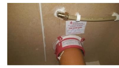
give rise to an opening that will allow significant fire and smoke spread. Proprietary fire seals, including externally-mounted collars, or fire-resisting enclosures, are used in new buildings and could be used to address this problem in older blocks. However, the difficulties of retrofitting such seals in an occupied block of flats may mean that it will only be practicable to undertake this on a long term basis as and when flats become vacant.
